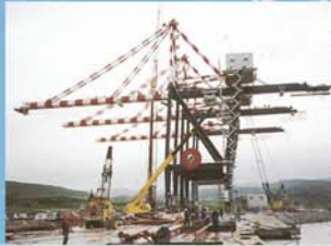
RMQC - Container cranes, Gioia Tauro, Italy 60 t x (50 + 20 + 16) m
